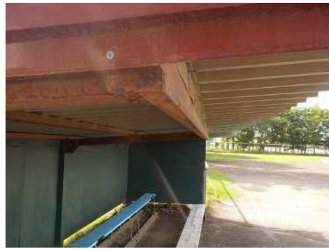
(三墨側腐食部)
